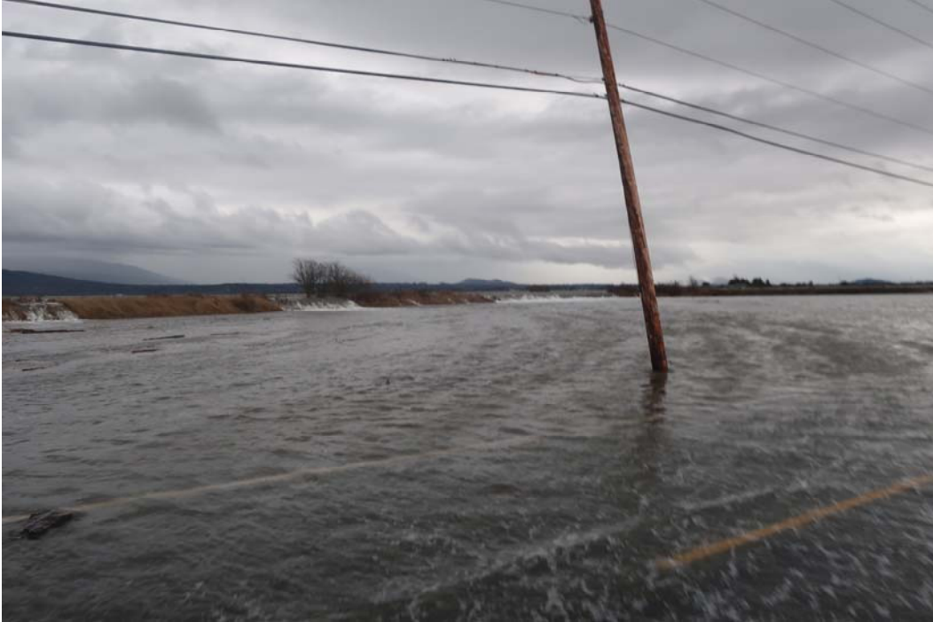
Tide water spilling over the dike and flowing across road during flood.
