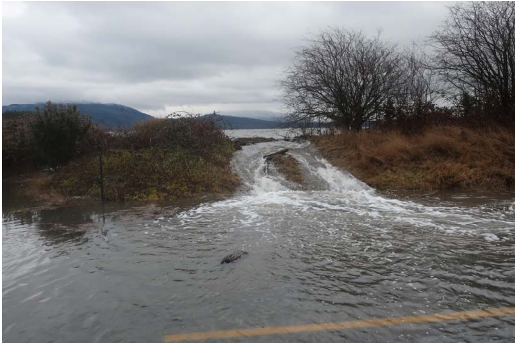
Water spilling over a northern section of dike adjacent to the road.
